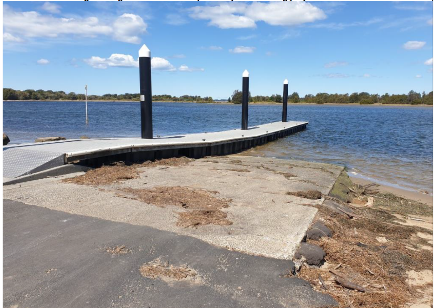
Photo 1. Site showing existing concrete boat ramp and adjacent floating jetty
